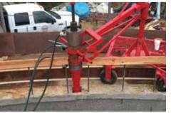
AWWA D110 Type I tanks incorporate vertical prestressing threadbars within the wall to provide vertical compression and counteract bending.
