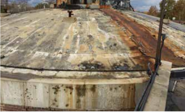
Before - Existing tank dome replacement
