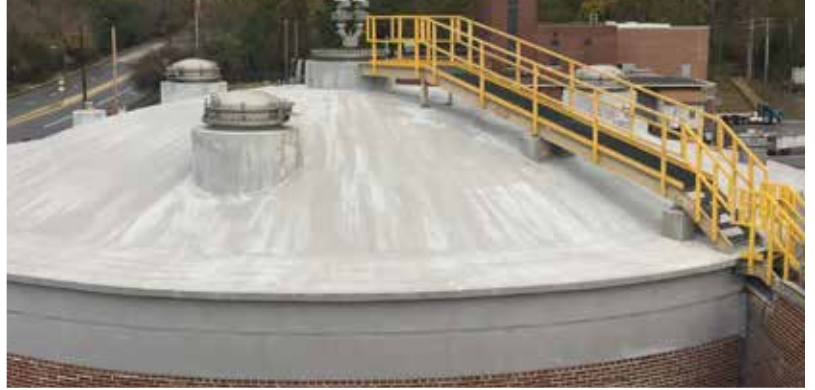
After - Existing tank dome replacement
